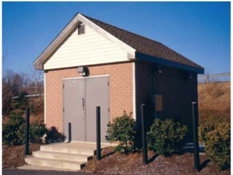
Generator building, Oliver City Sanitary Sewer System Warrenton, VA
