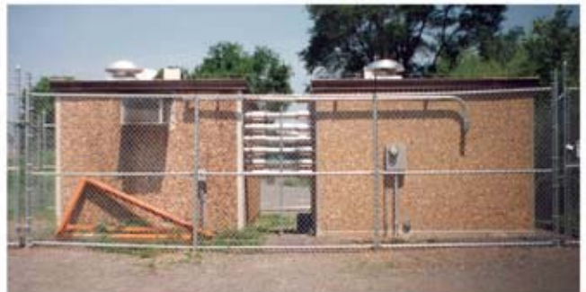
AT&T fiberoptic regeneration shelters, Calverton, VA
